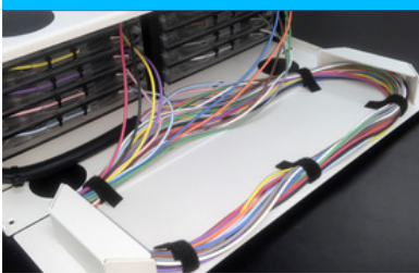
Built-in slack storage keeps fibers neat and manageable
